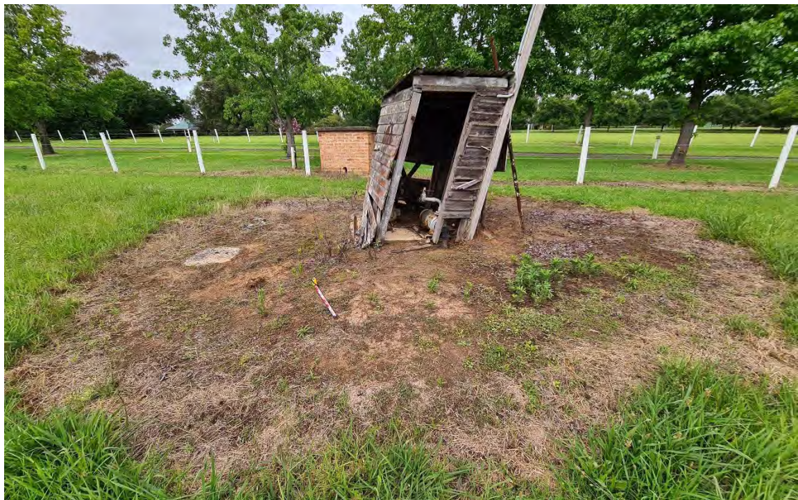
Figure 2.8 Area of exposure surrounding pump shed and utilities pole
